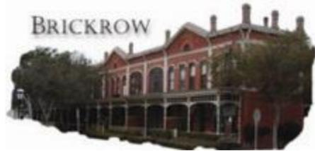
Twelve-inch thick interlocking brick walls divide the units. The brickwork on the row houses was laid with an artistic eye to break the severe lines of the long walls. The bricks above the second story are set upright at an angle. A one-story wooden porch runs the length of the building.
