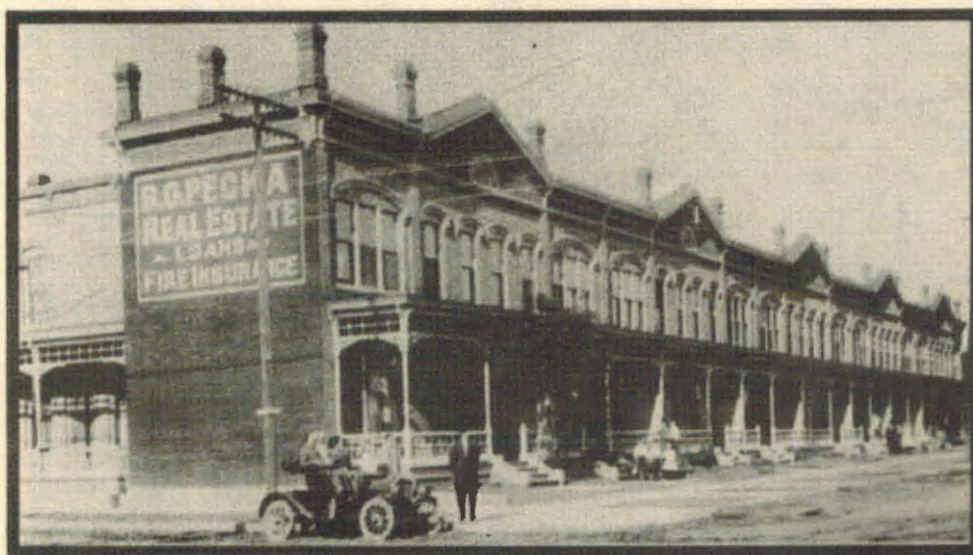
The Brick Row, around 1911; chimneys on the front of the structure were for decorative purposes.
